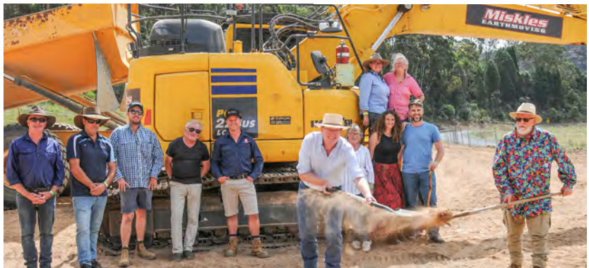
Construction of the Multipurpose Community and Relief Centre began on Saturday, February 24 when Federal MP Andrew Gee and Cox's Creek resident Bryan Ludwick turned the first sod. They were joined by local community members and Miskles Earthmoving staff for this historic moment.
