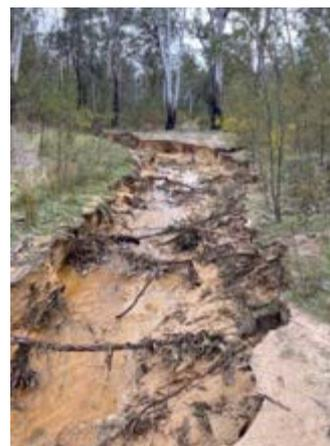
This property access road is completely washed out leaving owners isolated. It's the result of continuous rain events over many months leading to saturated ground that can't hold any more moisture.
