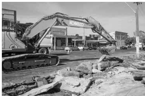
Making light work of huge slabs of concrete in Angus Avenue.
