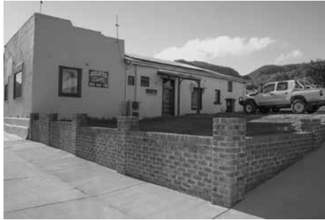
The new retaining wall at KRR
