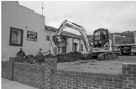
Early stages of work on new sewage line and retaining wall at KRR.
